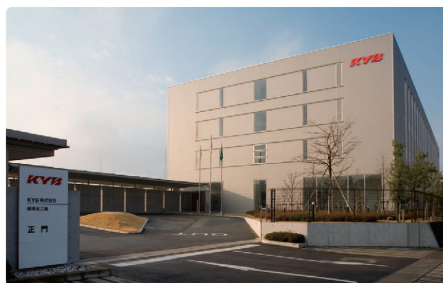
Gifu North Plant
